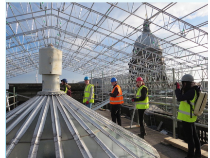
ECA students inspecting the roof of Old College on a unique educational trip to a live building site.
